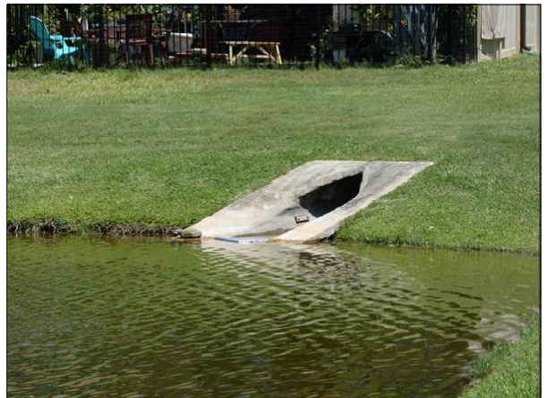
Stormwater Drainage Mitered End Section
