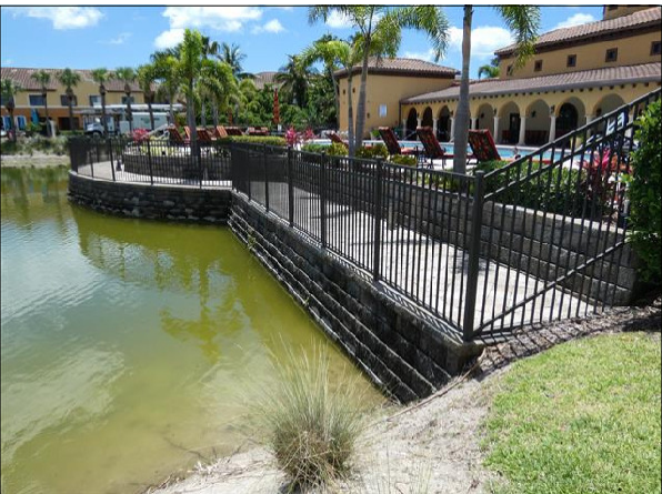
Retaining Wall at Clubhouse
