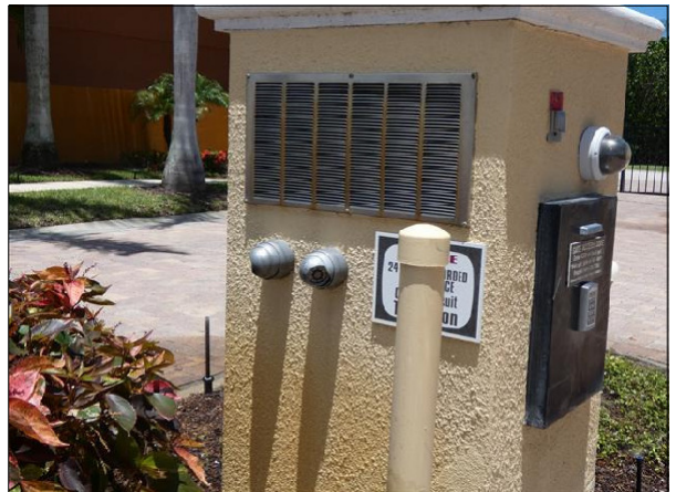
Security Camera System
