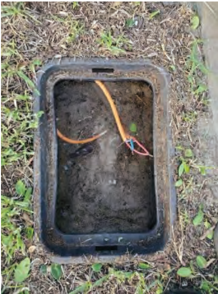
Missing wire nuts
