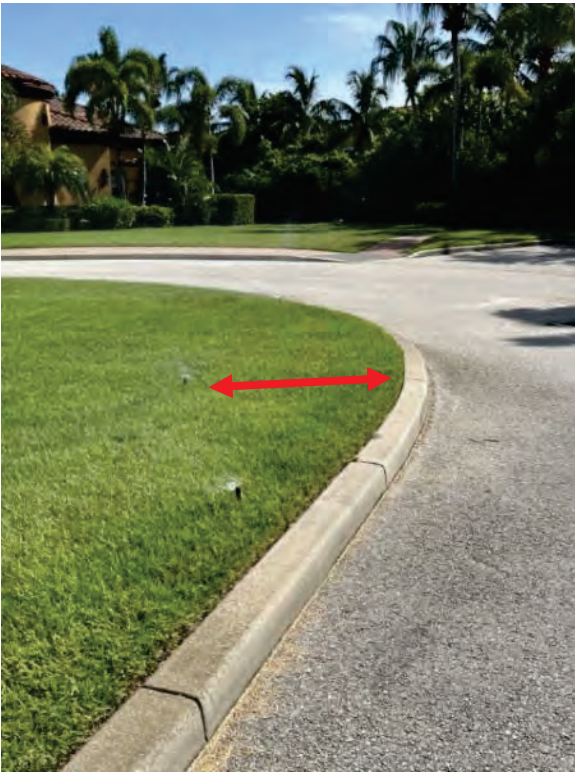
Irrigation head must be by the curb.
