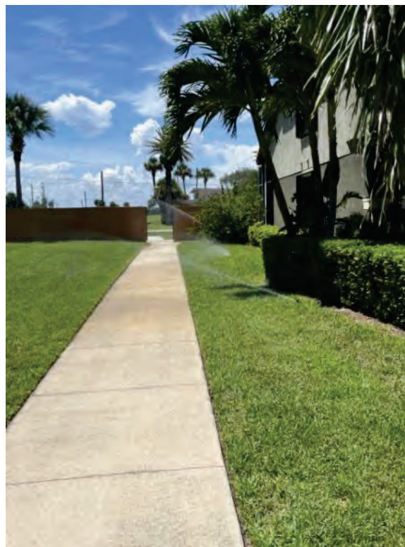
Heads spraying across the sidewalk
