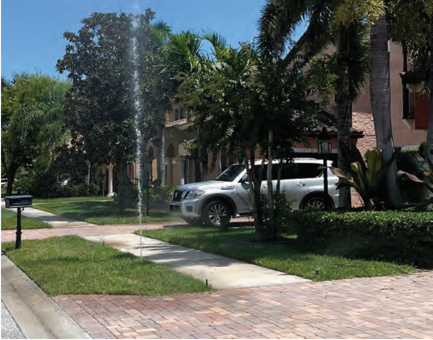
Broken head in August
