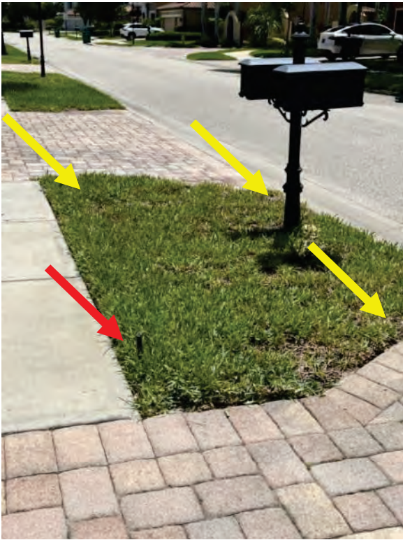
Clogged Nozzle and missing heads – notice turf
