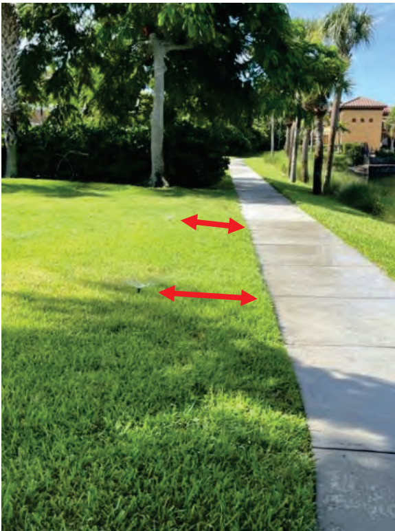
More alignment issues – the head needs to be by the curb.
