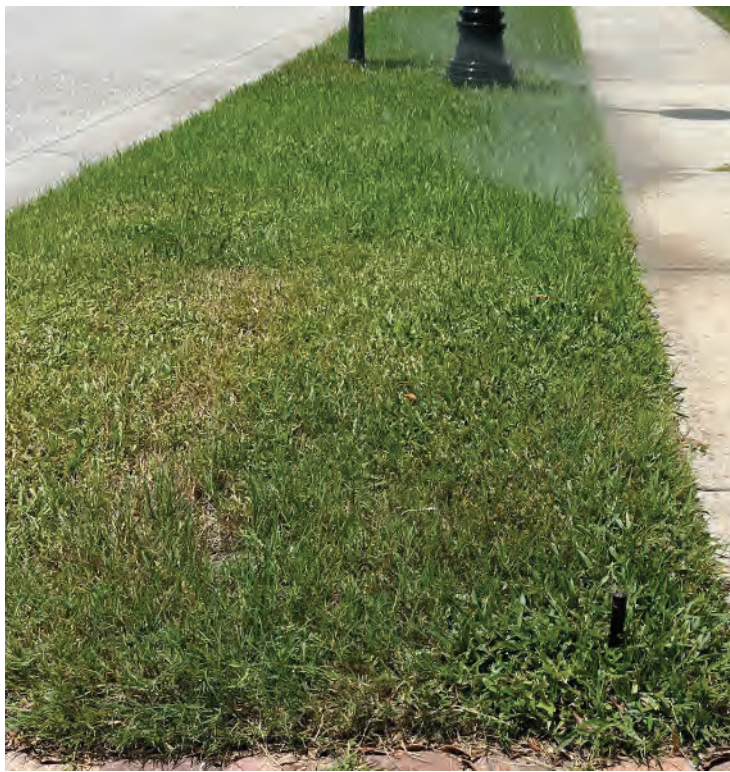
Tilted, too low, clogged nozzles
