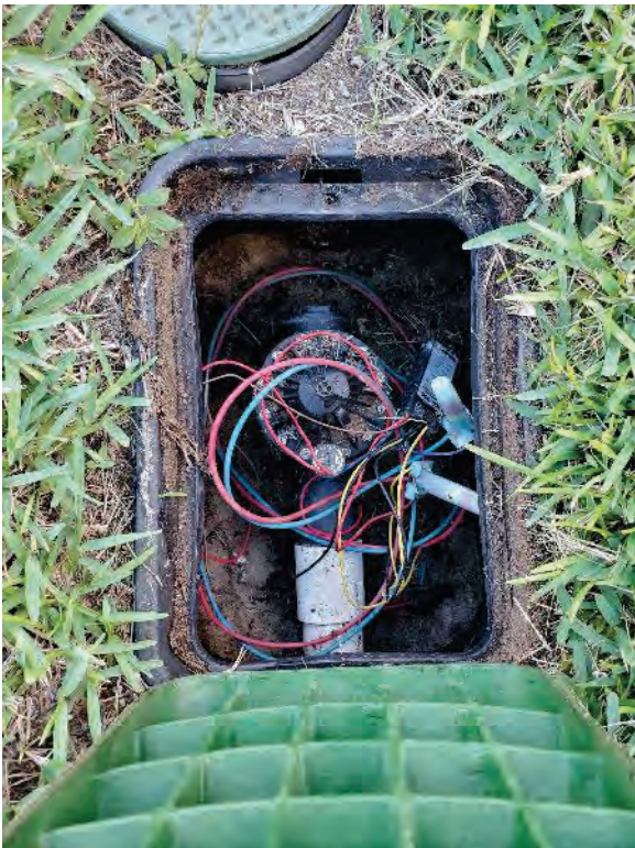
Valves boxes in relatively good condition
