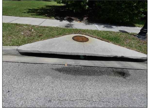
Stormwater Drainage Curb Inlet
