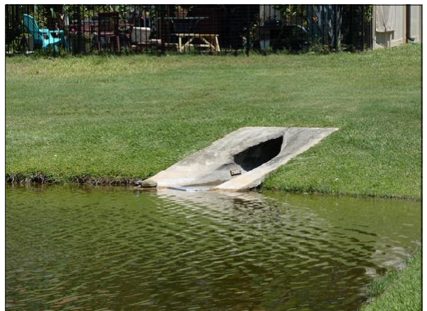
Stormwater Drainage Mitered End Section
